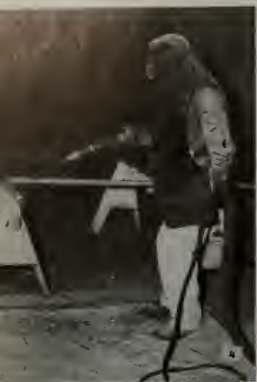
Fig. 4—Sandblasting is used on many operations in building tuna boats. Here, it is used for cleaning part of an ammonia coil for refrigerating system.
